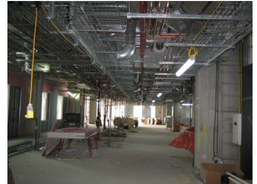
15/5/2009 Going down - ducting in place IMG_3949.jpg
